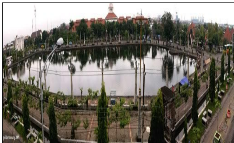
Figure 4 Tawang Retention Pond after completion in 2001.
