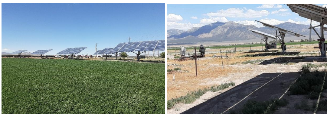
Figure 2. Dual Axis Sun-Tracking Solar Panel Systems for Irrigation and Net Metering in Central Utah
