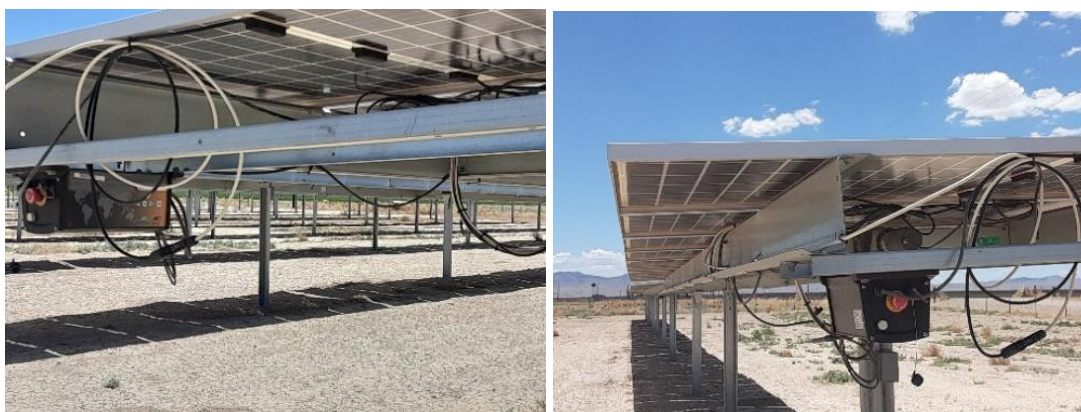
Figure 1. Single Axis Sun-Tracking Solar Panel Systems for Irrigation and Net Metering in Central Utah
