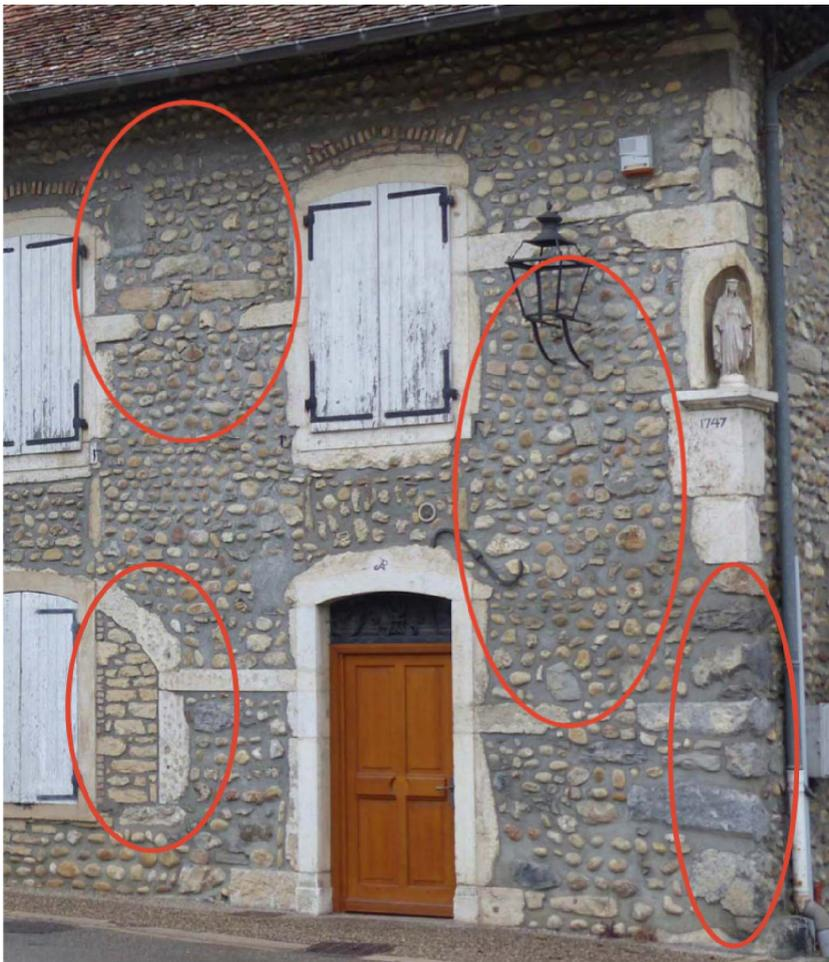
**Figure 6.** Damages and repairs observed for a masonry house (extracted from Poursoulis [2017]).
