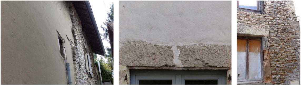
**Figure 5.** Examples of traces of damage in masonry structures: peeling of a wall, broken lintel, and crack in a wall (extracted from Poursoulis [2017]).
