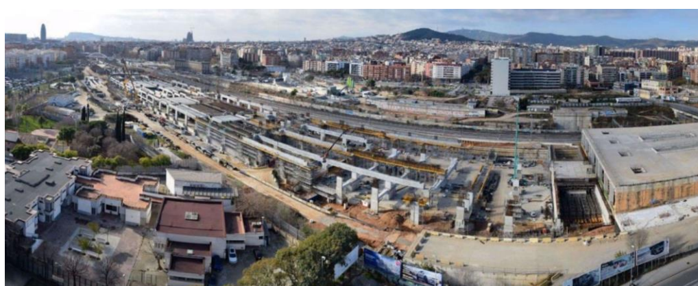
Figure 15 Construction of Ave in Sagrera (Barcelona)
