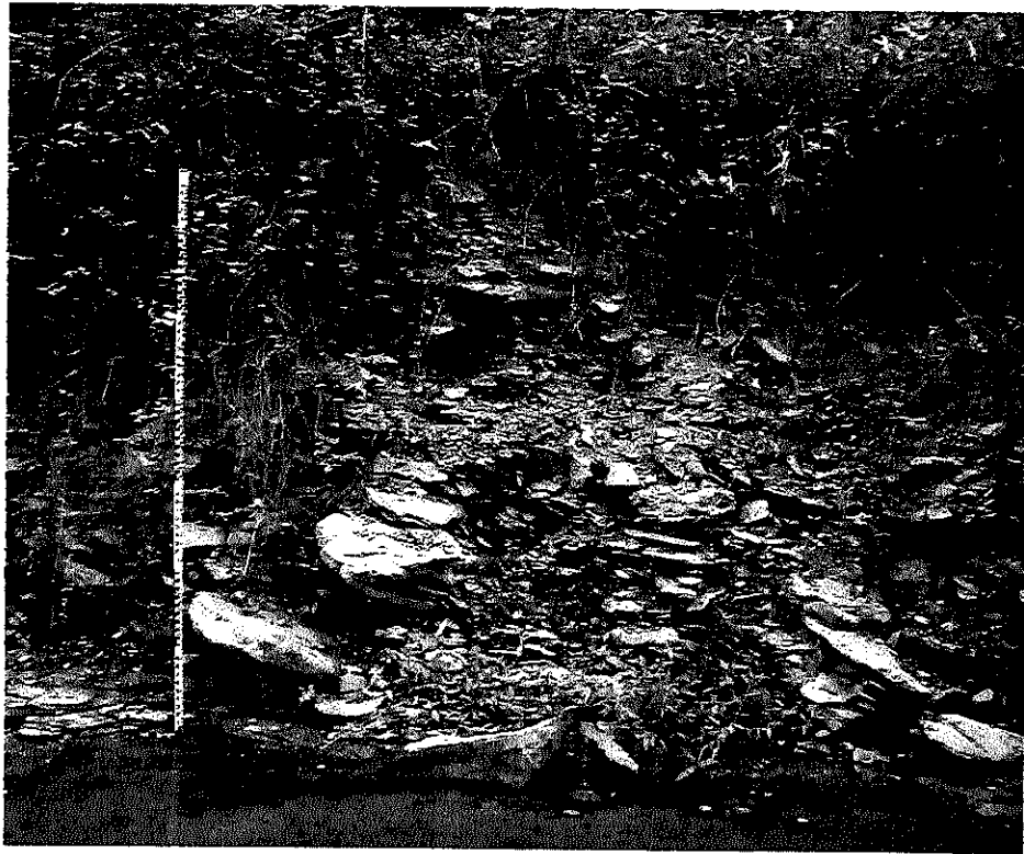
Figure 3.19. Eroded stream bank at Station 3+00 in Section 3 (bed rock) of Indian Creek.
