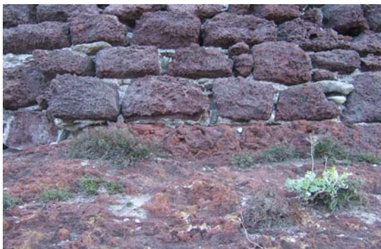
Fig. 3. The masonry made of volcanic rock blocks roughly shaped and put in place with an abundant mortar, made necessary by the irregularities of the same blocks
