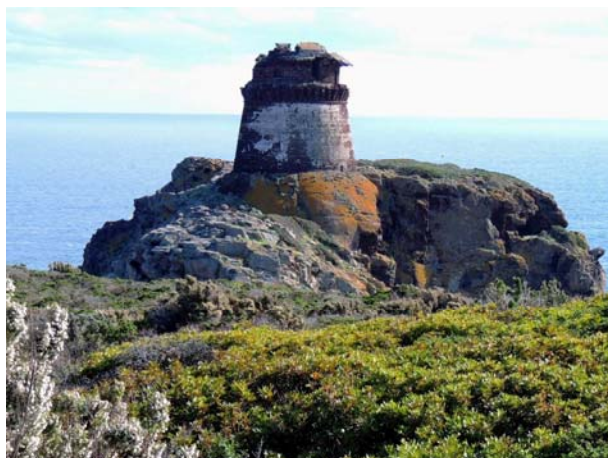
Fig. 2. The shape of the tower with the plastered conical base and the overlying cylindrical body with the corbels that supported a gallery
