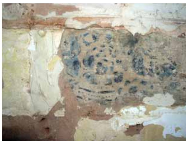
Figure 5: Paint scrape from house 3 evidence of 19 th century stencil wall painting.
