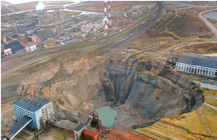
Fig.1. Sinkhole at the Uralkali mine (Perm Krai, Russia)
