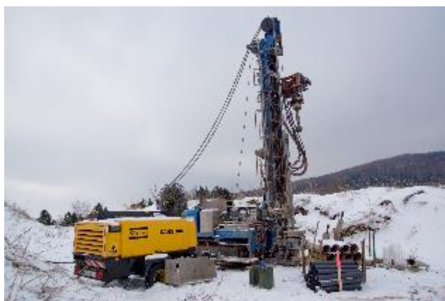
Figure 3: First drill campaign of project SMSB in Altenberg (TUBAF 2013)
