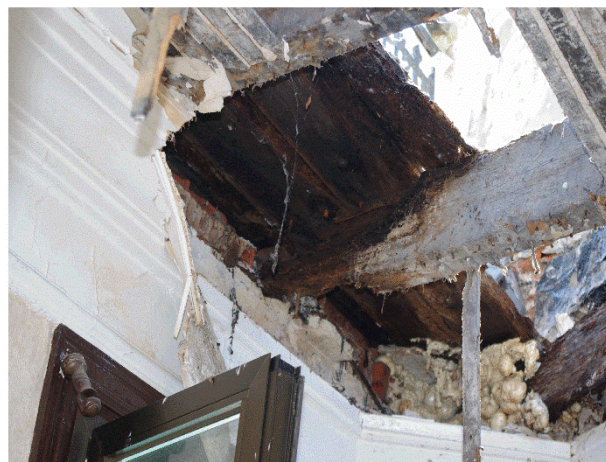
Figure 1. Wooden beam-end degradation sample in a self-evaluated case.
