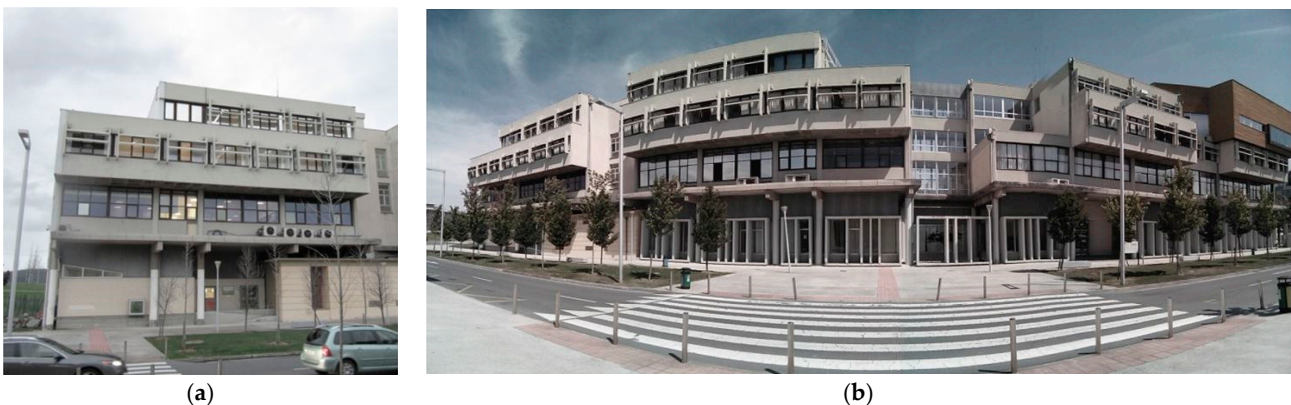
Figure 6. (a) The west block; (b) the southern view of the Rectorate building.
