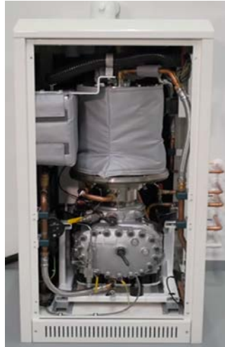
Figure 1.18 – Inspirit Charger micro-CHP system (Inspirit Energy, 2016).
