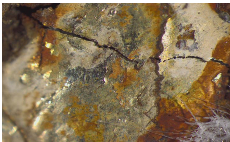
Figure 3.5: Detail of the gilded spur affected by degradation processes. In the image, cracks and swellings can be observed.
