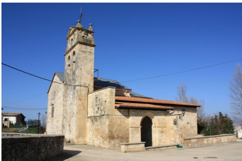
Figure 3.10: Church of the Assumption (Alaiza, Spain), external view.
