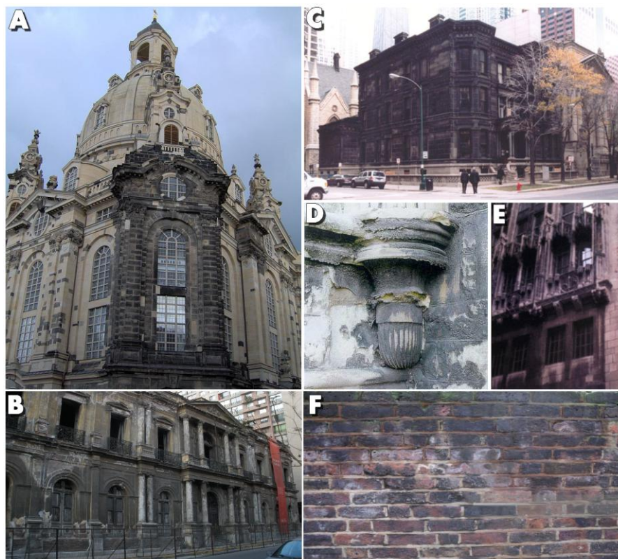
Figure 1.4. Examples of black crusts formed over A) limestone building surface in Germany, B) limestone building surface in Chile, C) sandstone building surface in U.S.A, D) limestone building corner surface in United Kingdom, E) sandstone building surface in France, F) brick wall.
