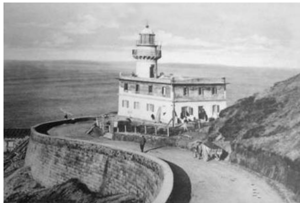
Figure 4.3. Historical photograph of Igueldo Lighthouse at the beginning of 20th century.
