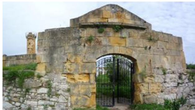
Figure 6.3. La Galea Fortress entrance arch.
