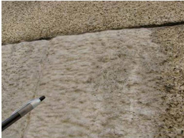
Figure 1.3. Example of white crust formed over building surface.
