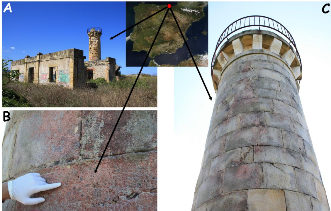
Figure 1. (A) General view of La Galea Fortress, (B) red biofilm colonizing the sandstone from the Northwest side of the Fortress tower and (C) general view of the Northwest side of the tower showing the red biofilm on the sandstone blocks.
