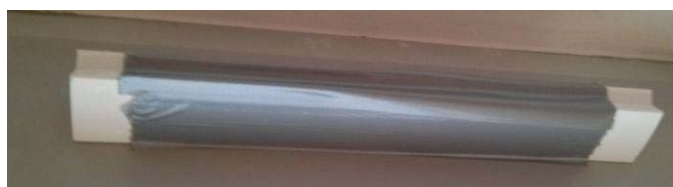
Fig. 4. 14. Sealing of ventilation grilles
