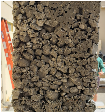
Figure 15: First pour: two lifts, no vibration, low water content
