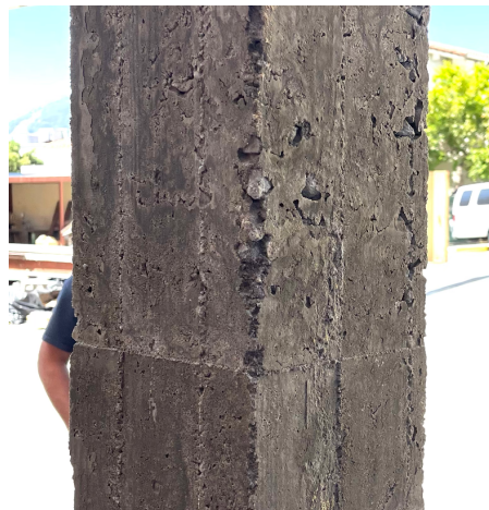
Figure 16: Second pour: one lift, trunk vibrator, higher water content
