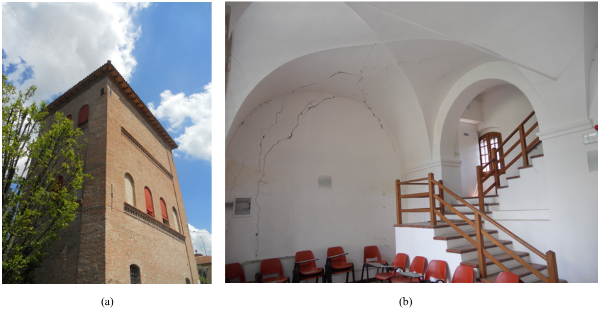
Figure 5: (a) External view and (b) first story masonry groin vault of Torre Fornasini (Poggio Renatico, Ferrara, Italy).
