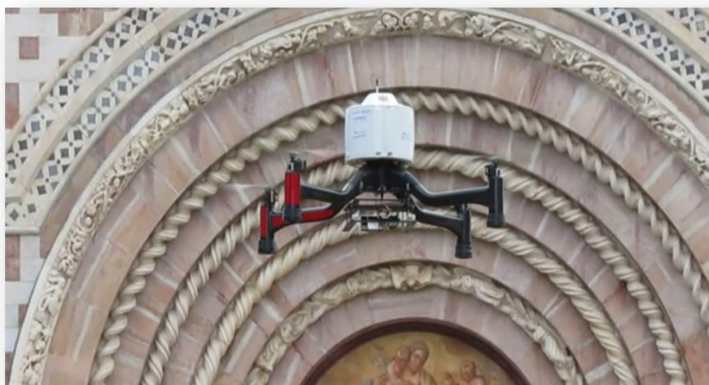
Figure 6. Quadcopter during the surveying of a facade during a post-seismic phase. Photo: M. Mormile (2015).
