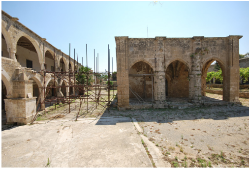
Figure 9 – The scaffolding is holding in place the leaning column, urgent intervention is required (photo: A. Camiz, 2014).
