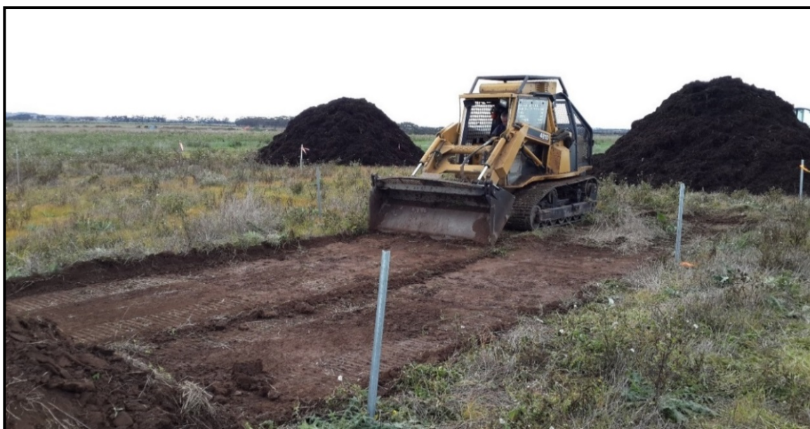
Figure 3.5 Topsoil removal (scalping) method.
