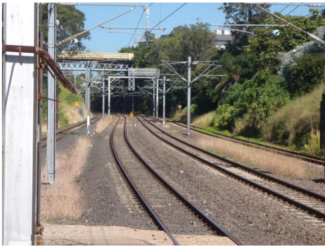
Figure 2. Safety issue in tight track access for maintenance crew [11]
