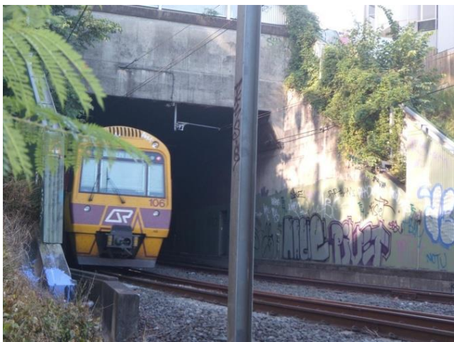
Figure 3. Access and safety issues for maintenance in tunnels [11]
