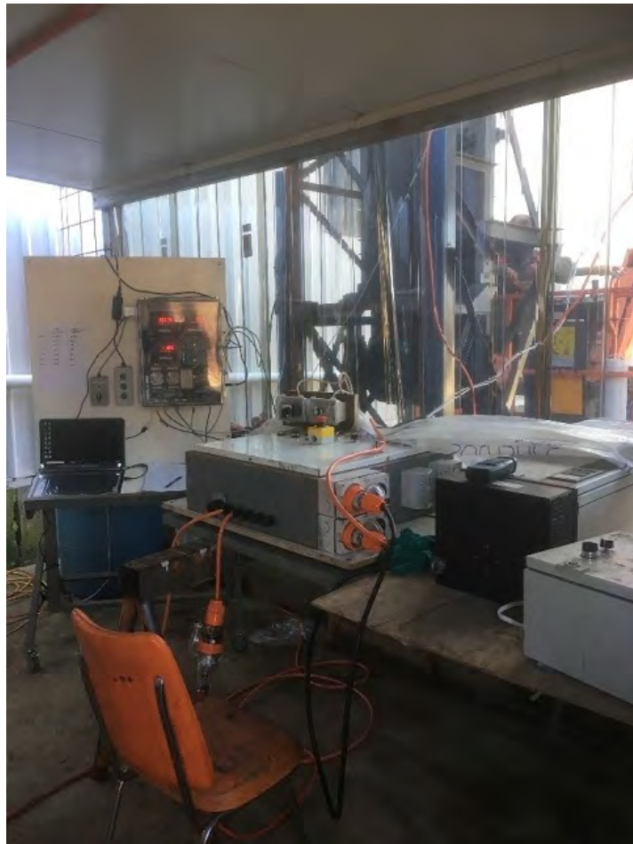
Picture 3A. Test Rig 3 control room showing the load cell weigh indicators and computer, the lower section of the hybrid elevator is partially visible through the window and in the foreground are the three VSD speed controllers for the cable disc elevator, the pipe conveyor and the ore bin discharge screw.
