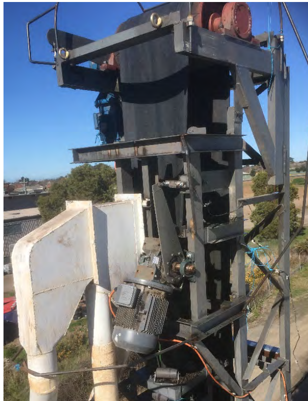
Picture 44 Test Rig 3 head drives with torque arms
