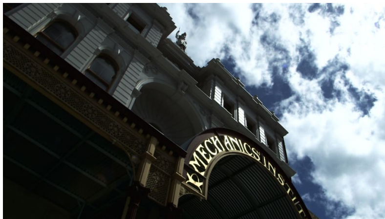
Figure 0.1: AVAT01 BMI building exterior, a still from 2016 promotional film Make Your Own History at the BMI produced by Yum Studio 2
