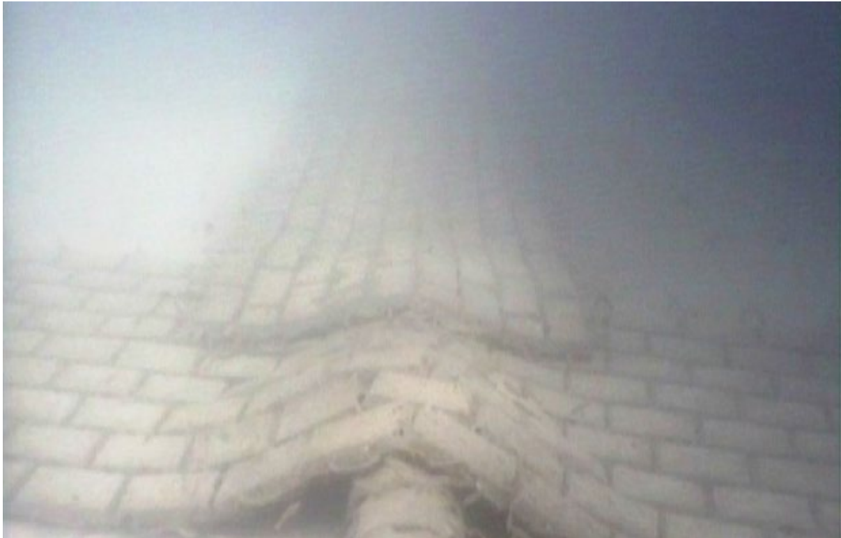
Figure 34: ROV survey showing the mattresses at the touch point.
