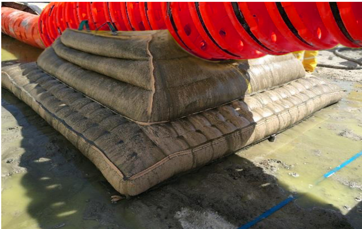
Figure 25: Mock-up trial for the cradle support
