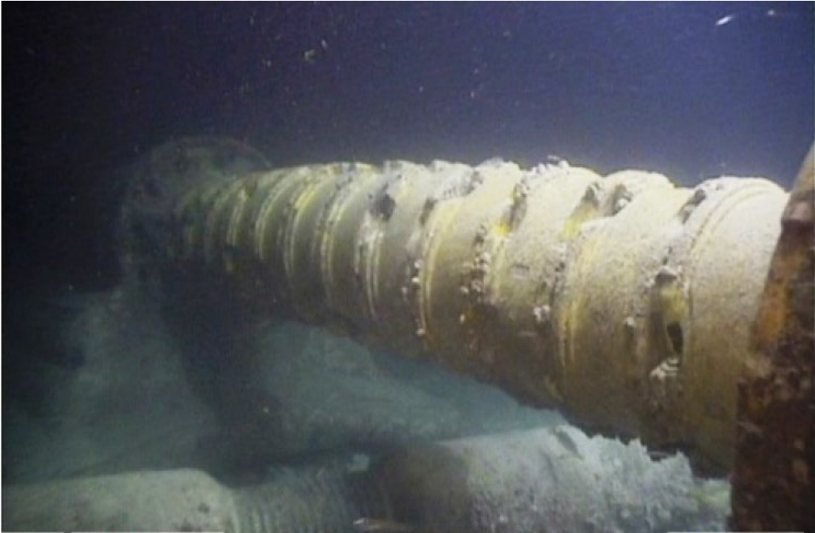
Figure 32: ROV survey for the cable and the bend restrictor
