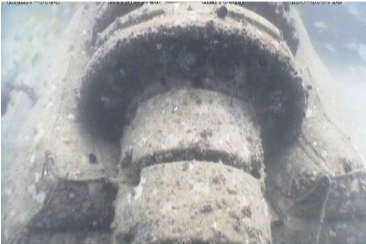
Figure 33: ROV survey for the cable and the cradle support.
