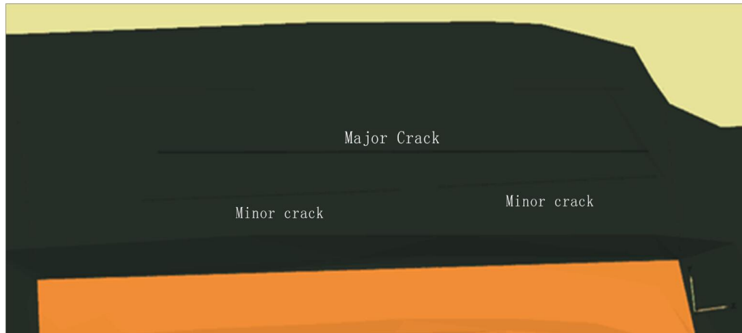
Figure 5.6 Aerial view of cracks on north batter surface
