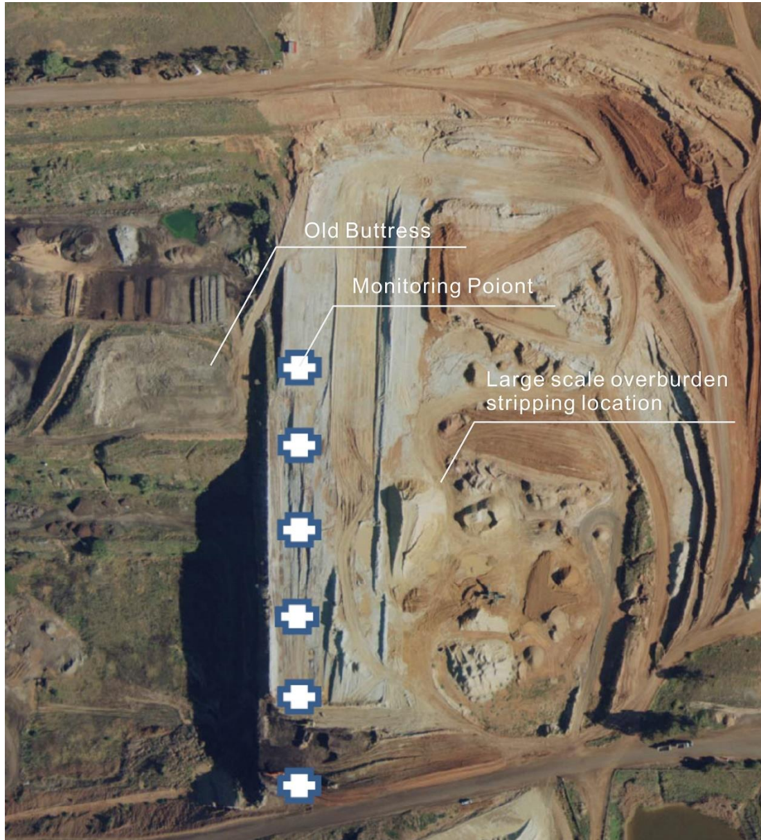
Figure 4.1 North batter coal face with the monitoring system established immediately after the observation of crack
