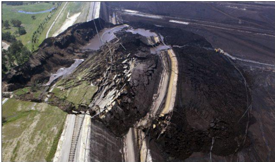
Figure 1.6 Yallourn batter sliding on 14th November 2017 (Petley, 2017)
