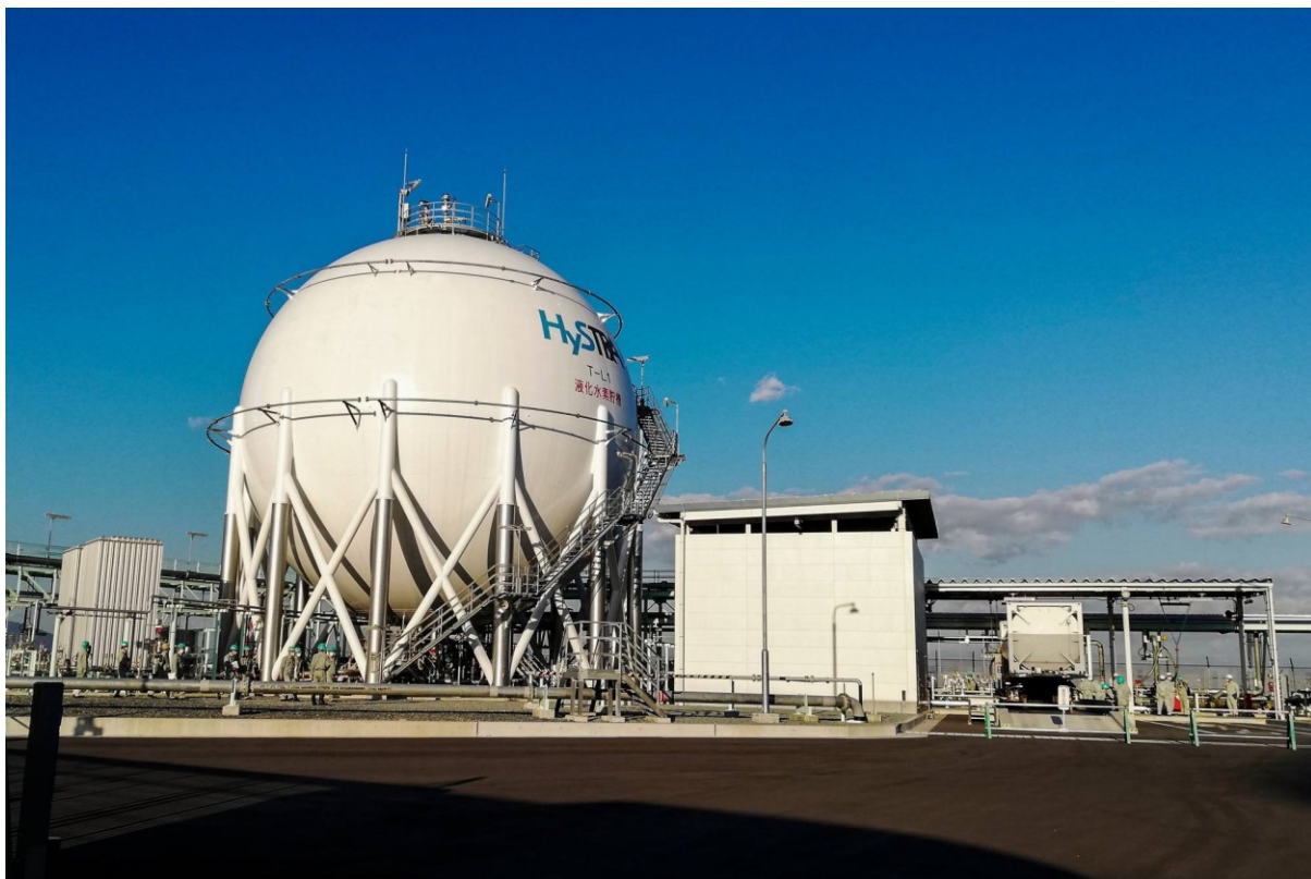
Figure 1.3: 2,500 m 3 LH 2 spherical storage tank built by Kawasaki on Kobe Airport Island, Japan. Reprinted from Japan Times, 2020. From https://www.japantimes.co.jp/news/2020/11/04/business/japanese-new-hydrogen-project/ .
