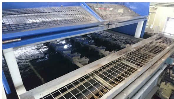
Figure 3-1 Waste activated sludge sampling from sludge thickening belt in WWTP1
