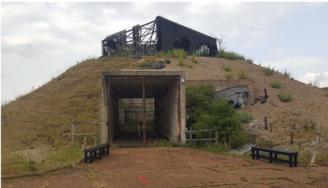
Figure 14: Outside the AWRE Laboratory 1 Building 2019
