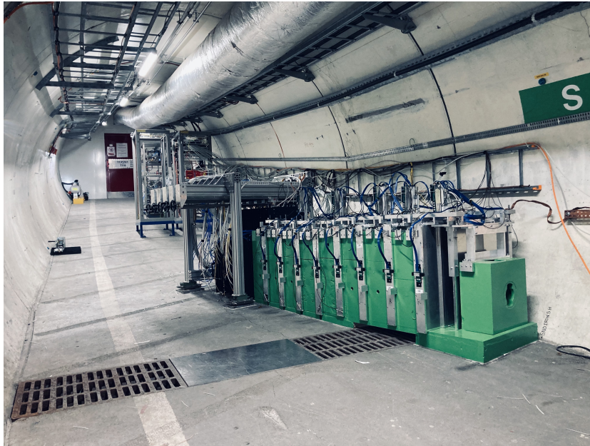
Figure 39. Side and top views of the SND@LHC detector in the TI18 tunnel.
