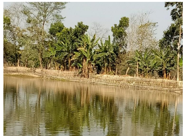
Dyke protection by erecting bamboo fencing (Nalbari)
