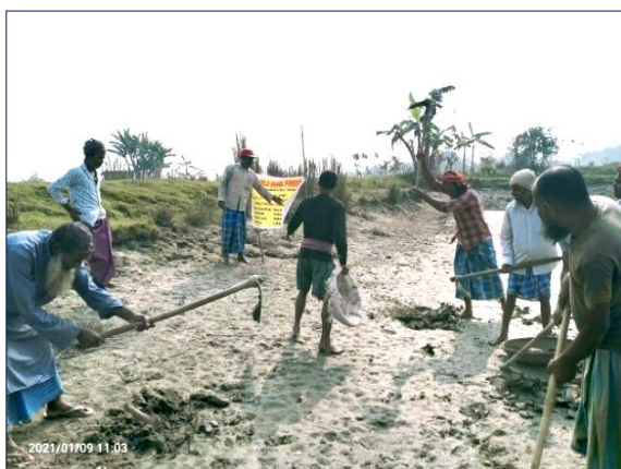
Land shaping work for paddy-fish integration
