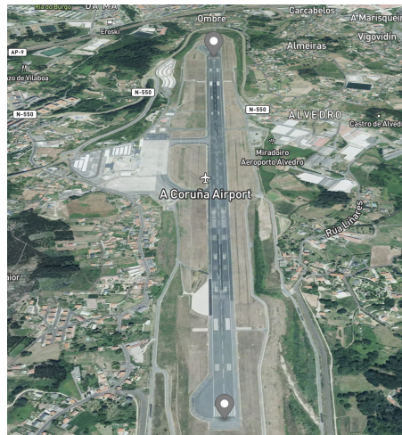
Figure 5.6: Coruna Airport Runways
