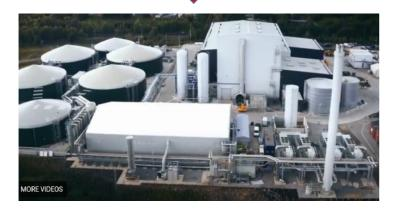
Production of biogas at 55°C and 15 days of hydraulic retention time
