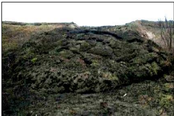
Figure 5 Landslide with muddy flow aspect
