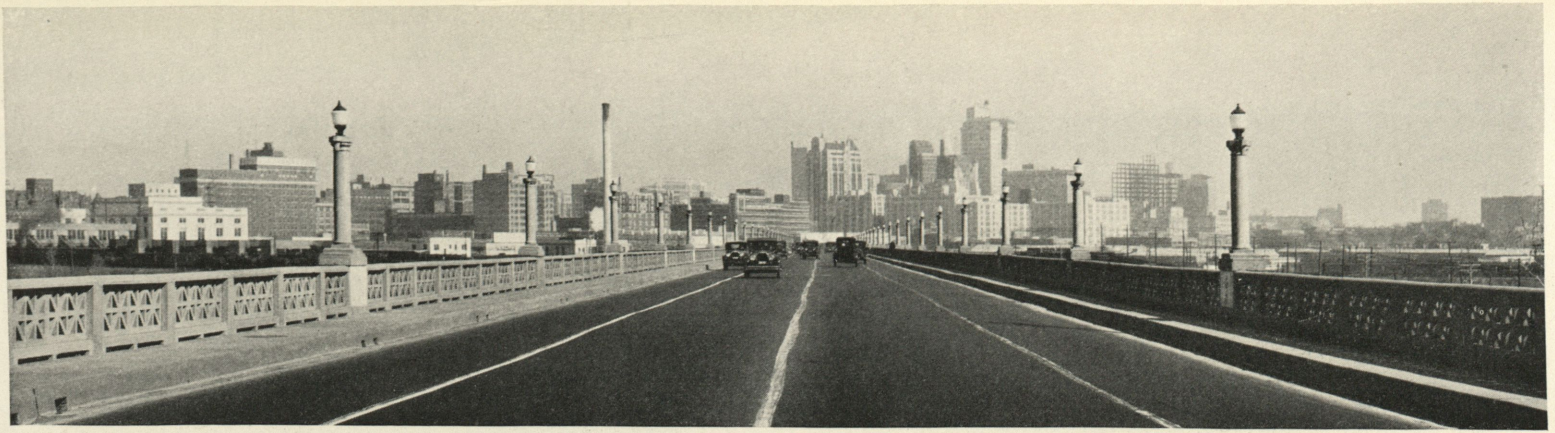
AS A GREAT DISTRIBUTING CENTER FOR THE SOUTHWEST, DALLAS RELIEVES THE TRAFFIC STRAIN ON ST. LOUIS AND KANSAS CITY Here literally scores of nationally known business enterprises have built warehouses. On busy days, over 200 package cars of goods leave Dallas for 11,000,000 consumers who live within a radius of 300 miles. This recently completed viaduct is more than a mile long.
