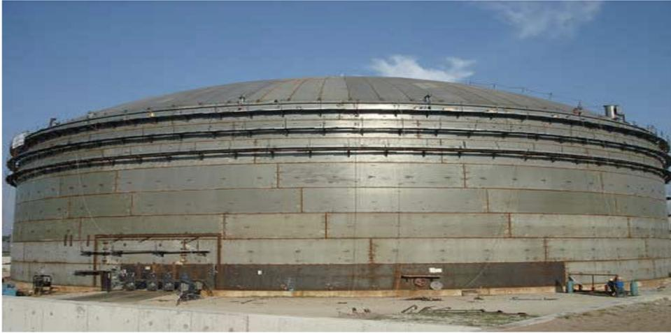
Figure 5.3: Internal floating roof tank
