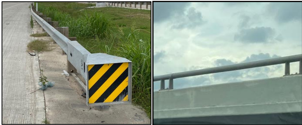
Figure 2 Typical roadside safety devices in Texas
