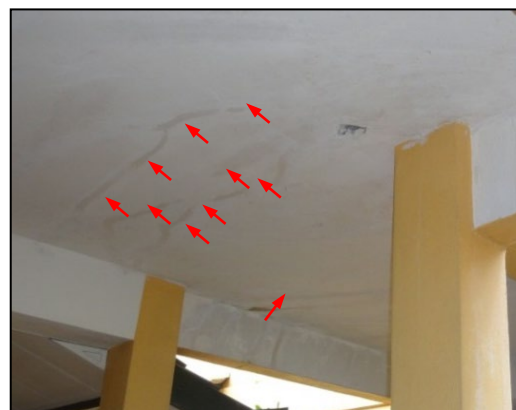
Sealed slab (photo was taken from the 1 st floor)
