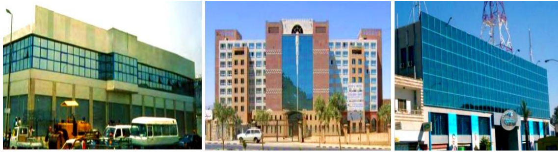
Fig. 9 - Contemporary buildings in Yemen
