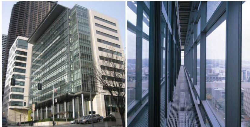
Fig. 1 - Seattle Justice Centre: example of double-skin façade [15]
