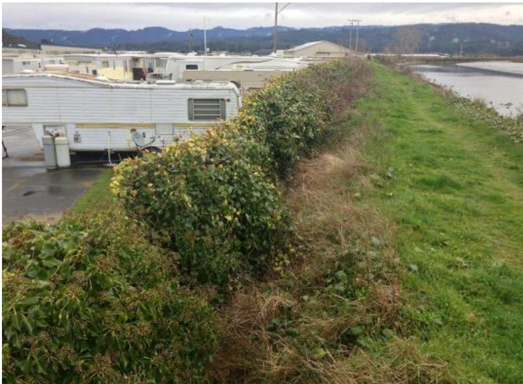
Figure 8. A photograph taken from atop Jacobs Avenue levee depicting the Lazy J mobile home complex below the levee top and the Eureka Slough separated to the right (south) (photograph by Evan Wisheropp).
