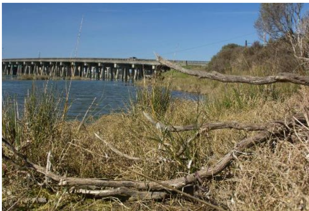
Figure 12. Photograph of the tract’s coastal wetlands while facing Eureka Slough Bridge at low tide (photograph by Evan Wisheropp).
