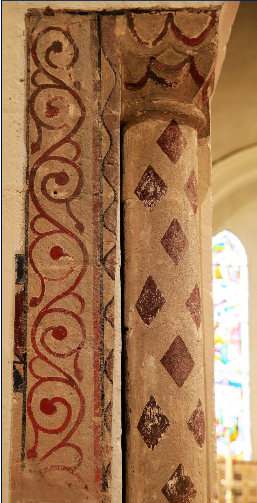
69 Cowley, chancel arch, N jamb.
