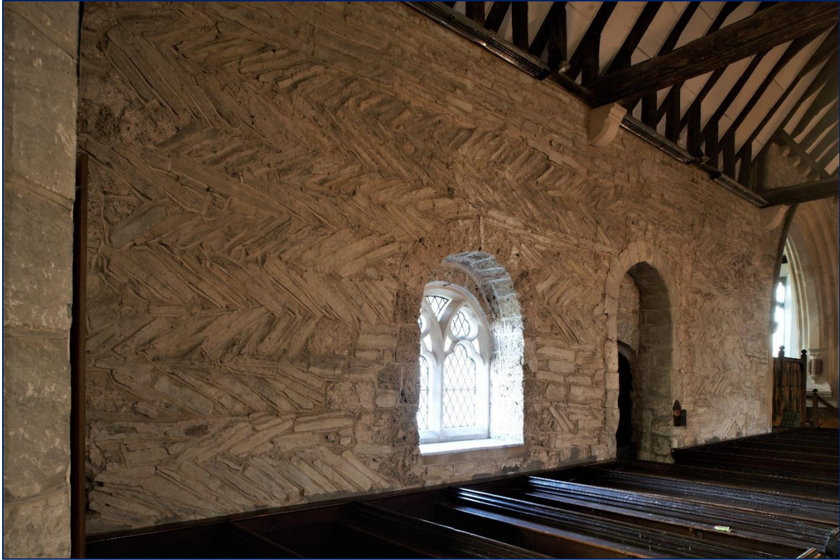
48 Ashleworth (Gloucestershire), St Andrew and St Bartholomew, interior, nave N wall, herringbone masonry for comparison with #47.
