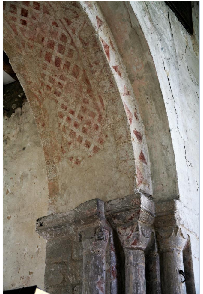
54 Duxford (Cambridgeshire), St John, W arch of central axial tower.
