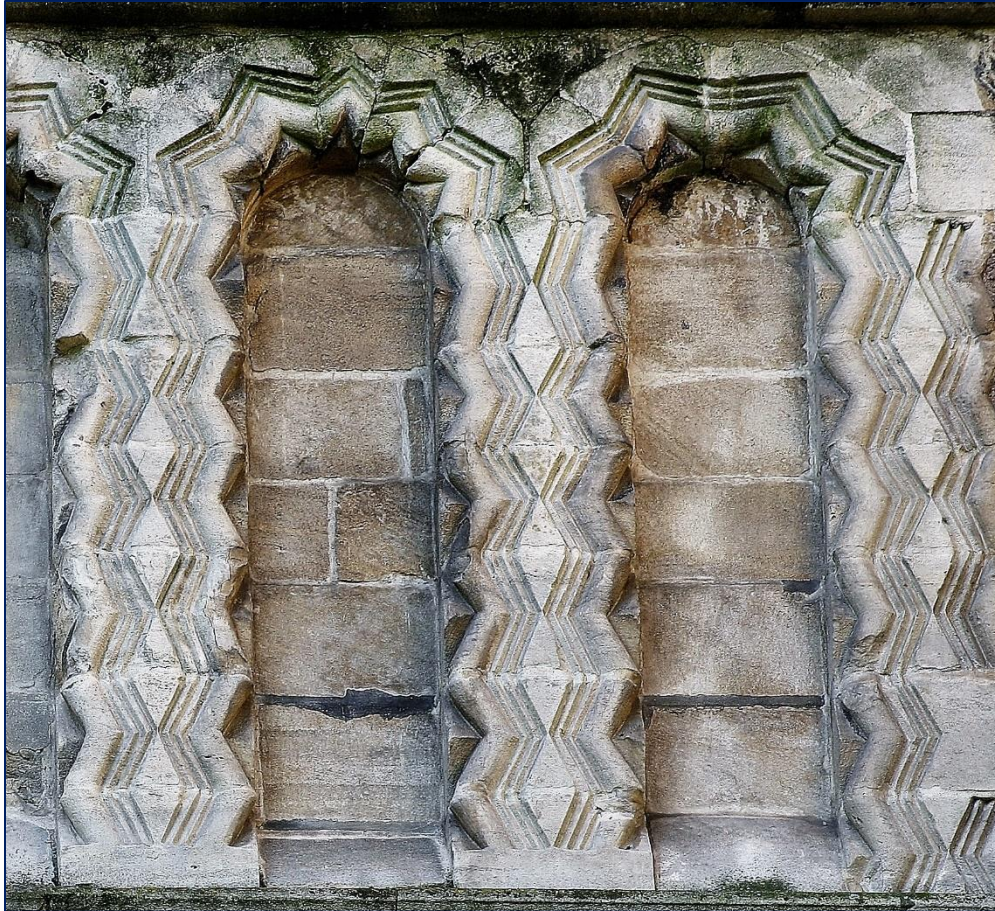
35. Gloucester. St Peter's Abbey, 'bridge' from presbytery gallery to W gallery of the Lady Chapel, reused chevron for family resemblance in chevron pattern with the painted work at Leominster, and the next two images.
