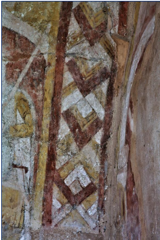
25. Kempley, Old St Mary's chancel vault, E end, chevron ornament, also used at the W end of the barrel vault. A complex three-dimensional variant of chevron which should be seen alongside contemporary patterns in carved chevron as in the crossing of Hereford Cathedral in the next image.
