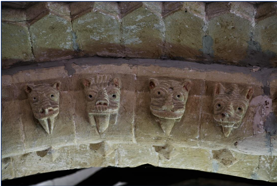
63 Avington, detail of #62. 11
