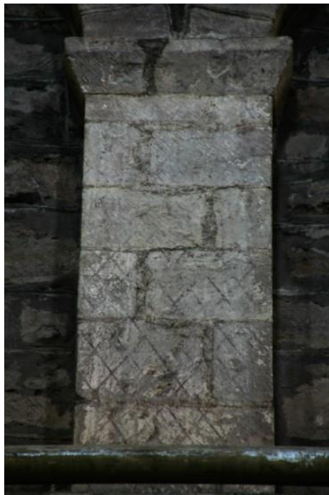
37. Hereford Cathedral, nave arcade detail.
