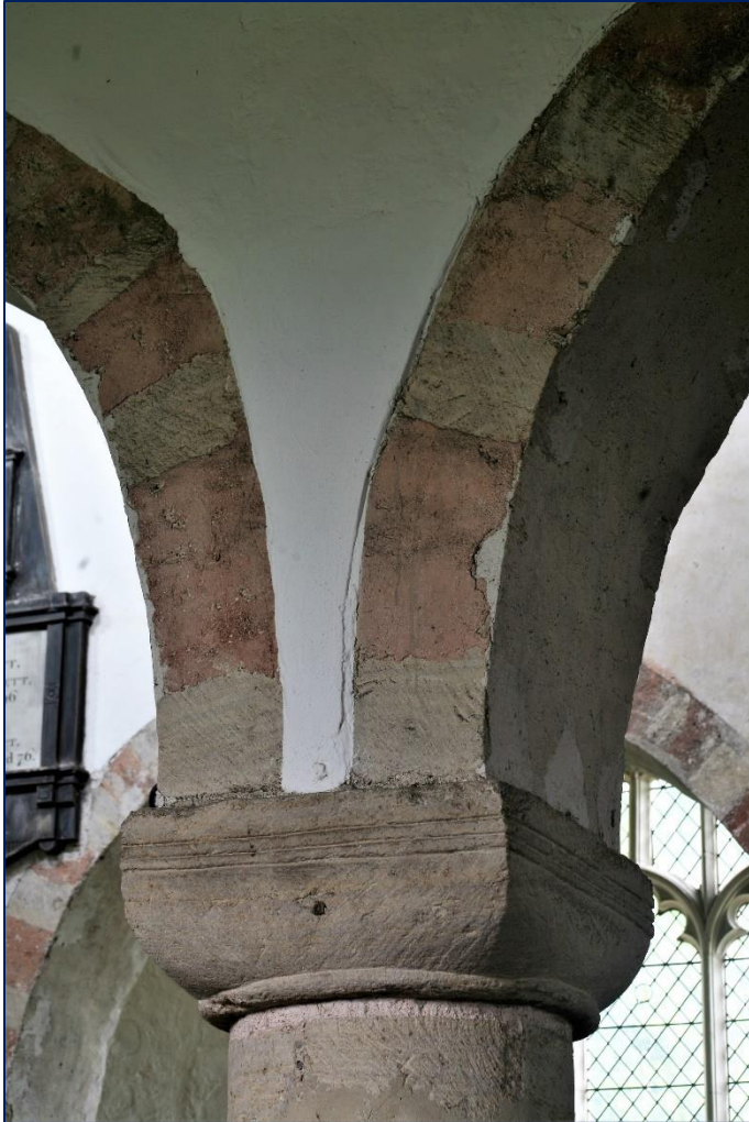
53 Ickleton, S nave arcade, detail of red fictive voussoirs recalling Roman practice of alternation brick and stone voussoirs as in Constantine's Baths at Trier.
