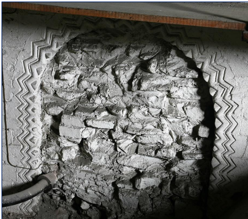
36 Hereford Cathedral, S transept E wall, blocked clerestory window from above high vault.
