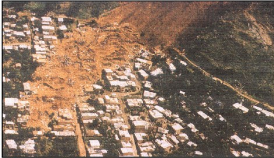
Figure 1: In 1987 a landslide in Villa Vallantina, Medellín, caused appr. 500 casualties triggered by a leakage at a water pipeline. Ojeda 2006, p.10.
