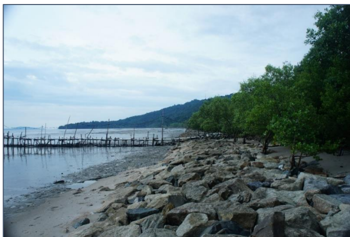
Figure 4.10: Rock revetments extended from the breakwater to the shoreline.
