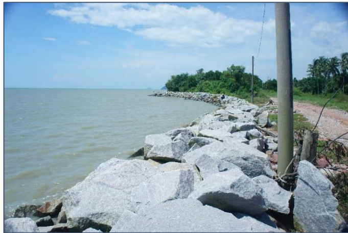
Figure 4.20: Rock revetments installed on the coastline as protection.
