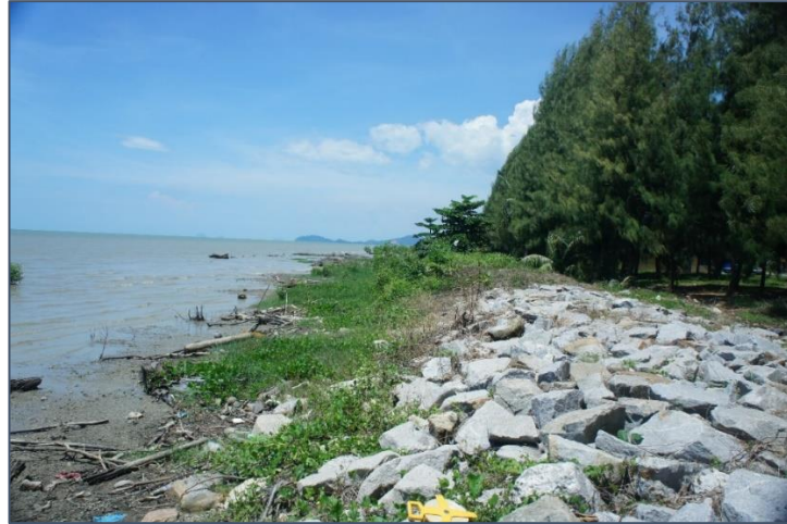
Figure 4.2: Existing rock revetments protecting Kota Kuala Muda from wave actions.
