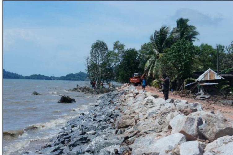
Figure 4.8: Recently constructed rock revetments to protect the coastline.
