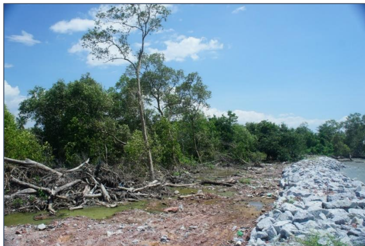
Figure 4.5: Constructed rock revetment to protect the shoreline from wave actions.
