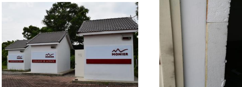
Figure 3-11 Experimental houses & wall of experimental houses that installed with 100mm thick Styrofoam in Monier Sdn Bhd, Shah Alam.
