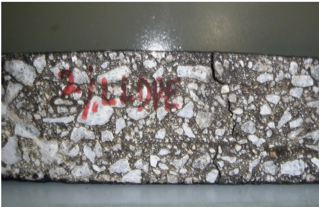
Figure 17: Crack Pattern observed for 2% LLDPE PMB Bituminous mixture beam
