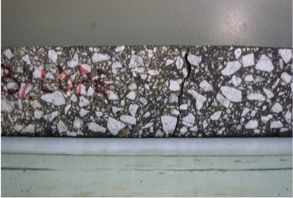
Figure 18: Crack Pattern observed for 3% LLDPE PMB Bituminous mixture beam
