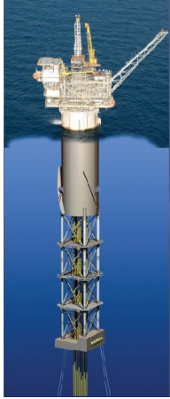
Figure 1.1: Truss spar platform
