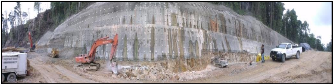
Figure 3.3: Overview of “Slope A”
