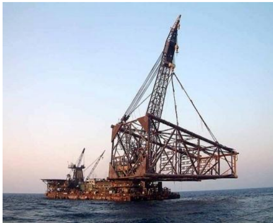
Figure 2. 3 Removal of Jacket Platform
