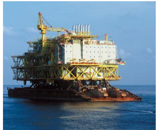
Figure 2. 4 Transportation of Topside to Scrapping Yard
