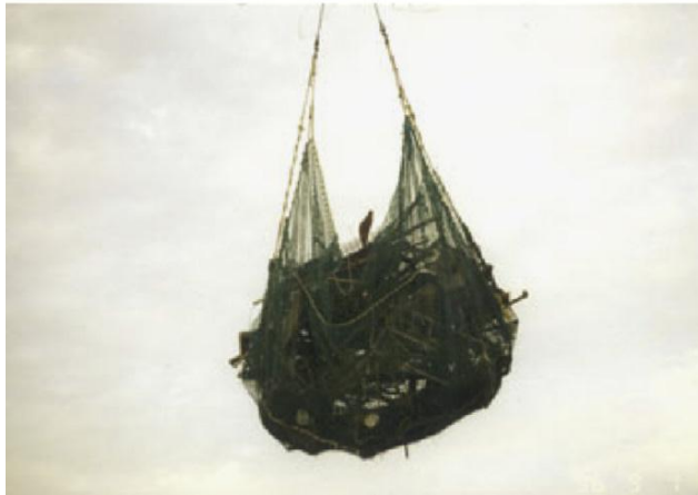
Figure 2. 5 Net Trawling Technique for Site Clearance
