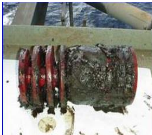
Figure 2.10: The scrapper coated with wax in Nigeria pipelines
