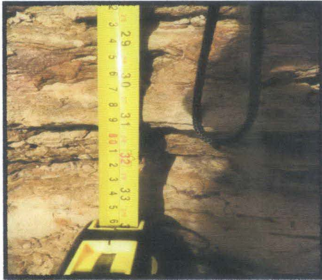
Figure 3A Measurement of thickness using measurement tape
