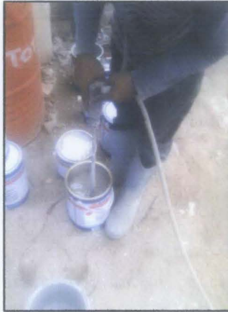
Coating preparation process – mixing and stirring
